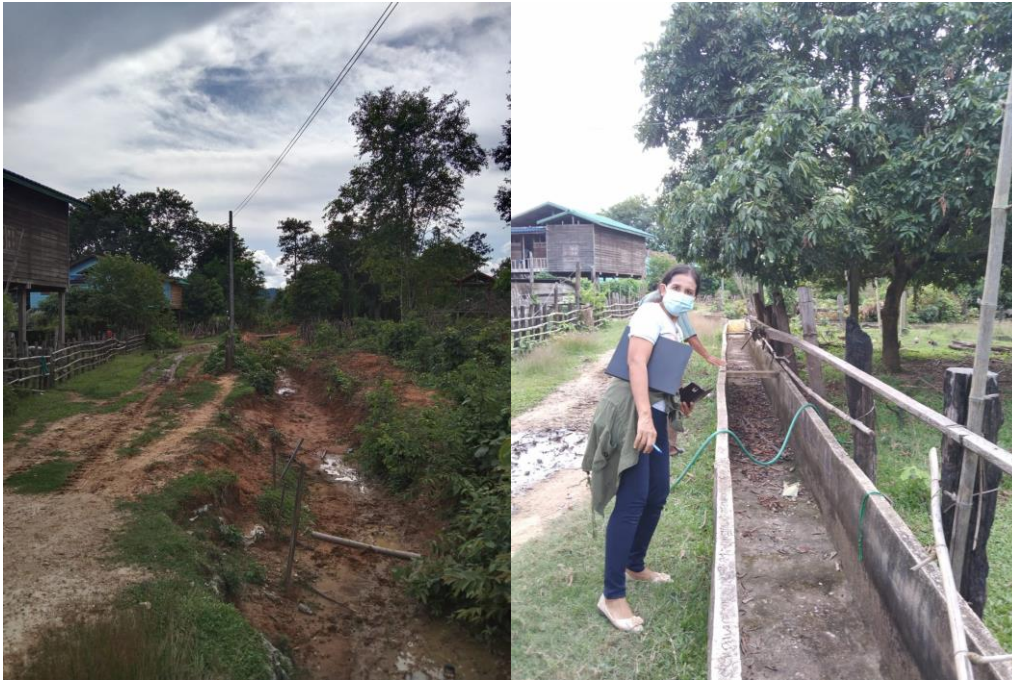
Figure 3. Existing and Proposed Main Canal Construction Extension
